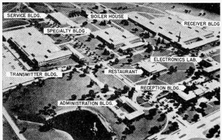
ELECTRONICS PARK, the twenty-five million dollar manufacturing and research centre of General Electric at Syracuse, N.Y.
